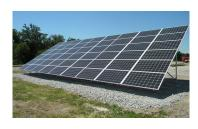
Two ground-mounted solar photovoltaic systems were built in June 2015 at the Secondary Roads/ SEATS campus. By mid-summer, once electrical hookups are in place, the panels will generate nearly 86 kW of energy each year for the Secondary Roads Shop and West Garage.
