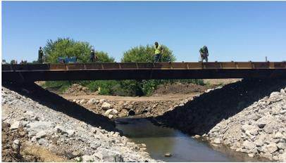
The Secondary Roads Department repurposed three railroad flatcars into a strong bridge for Lower West Branch Road, keeping an estimated 100,000 pounds of steel out of the scrap yard. The department also used 923 tons of recycled materials to pave Wapsi Avenue,
