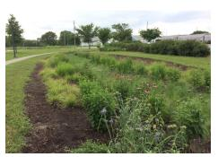
The bioretention cell near the Administration Building saw refreshed soil and plantings in 2017. By spring 2018, 12 varieties of flowers and grasses were thriving. The cell slows and filters stormwater—an important function in urban areas where concrete makes many surfaces impervious to water.
