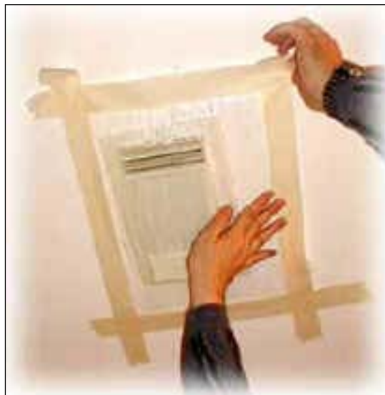
Sealing an Air Vent
