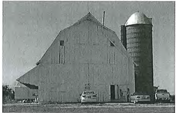
DAIRY BARN, Johnson County Poor Farm, IA (7/2013)
