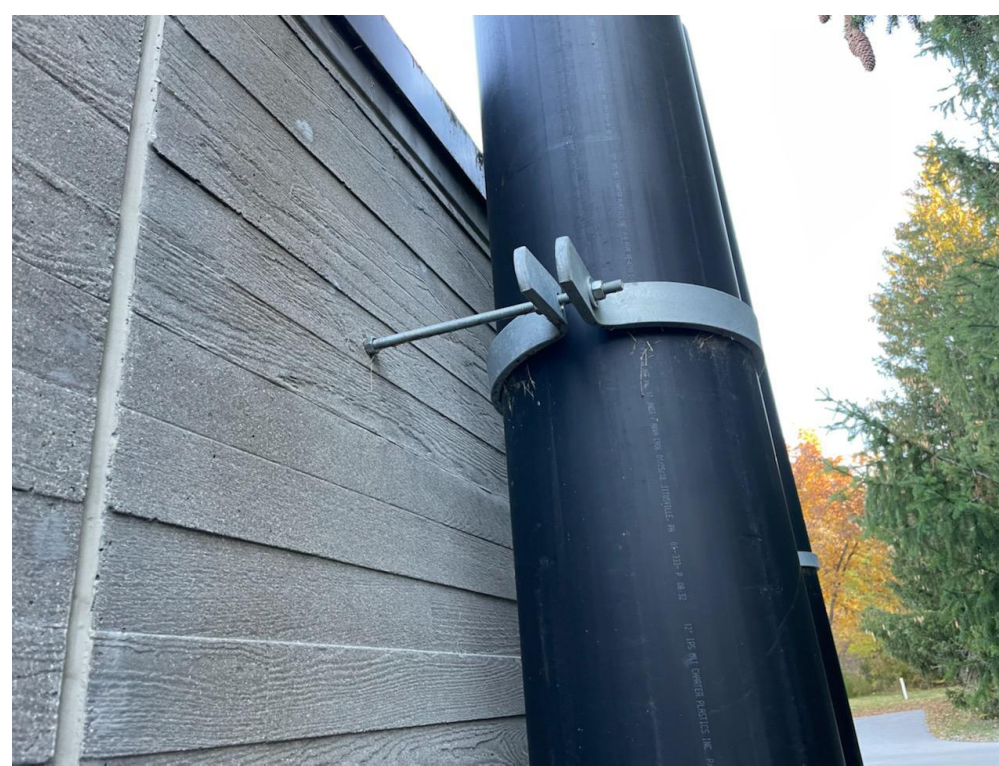
6 VENT STACK BRACKET 1 1/2" = 1'-0"
