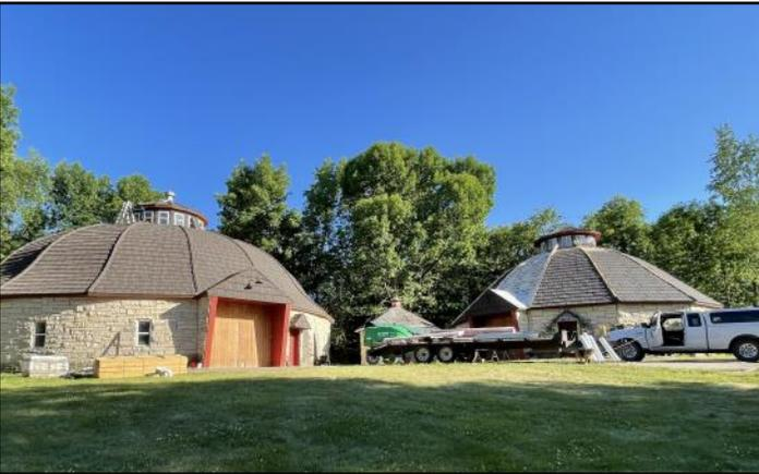
The roofs on 5 barns at Cangleska Wakan were damaged by the derecho and work began on re-shingling 4 of them during the fiscal year. In addition to the barn roofs, the barn doors sustained damage when they were inverted from the high winds, a lean-to at the site was destroyed and the high-tunnel used for production of local foods was damaged.
