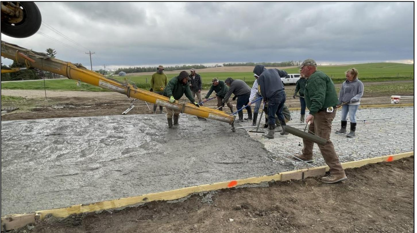
May 6, 2021. The Operations and Maintenance staff pour the concrete entry drive at the new Sutliff Operations Center. The project took three days to pour and saved the county approximately \$85,000 by doing it in-house.
