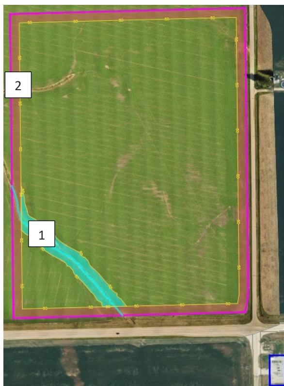
Figure 4. Plot Areas of the Lone Tree PV Plant
