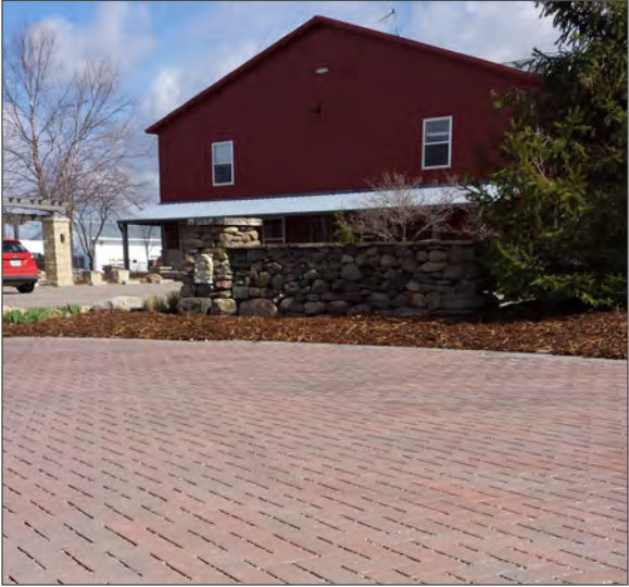
LEFT: An example of permeable pavement, which helps reduce stormwater runoff. RIGHT: Cover crops can help reduce soil erosion and contribute to soil health.
