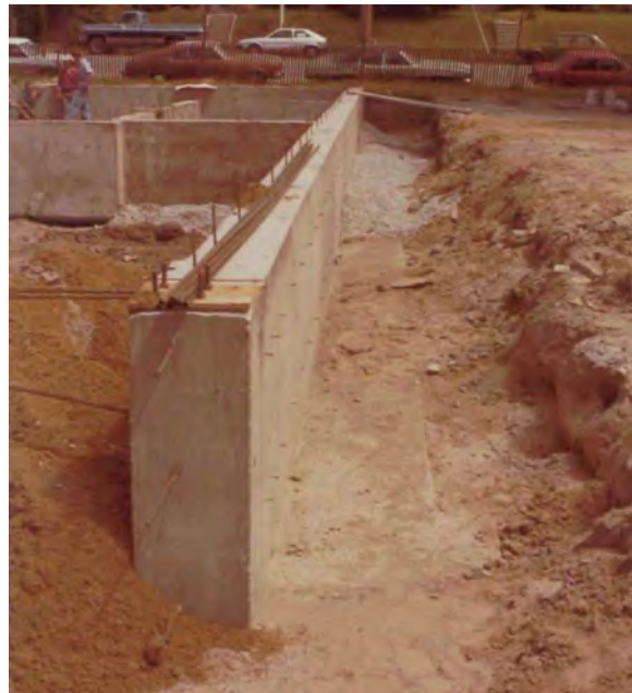
CIP PCC foundation and footing
