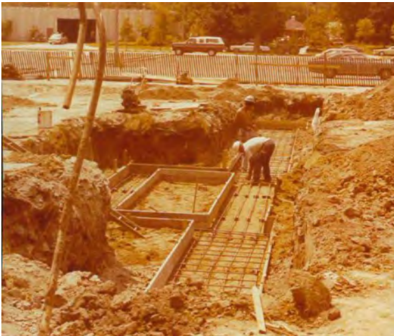
1979 photo of footing construction
