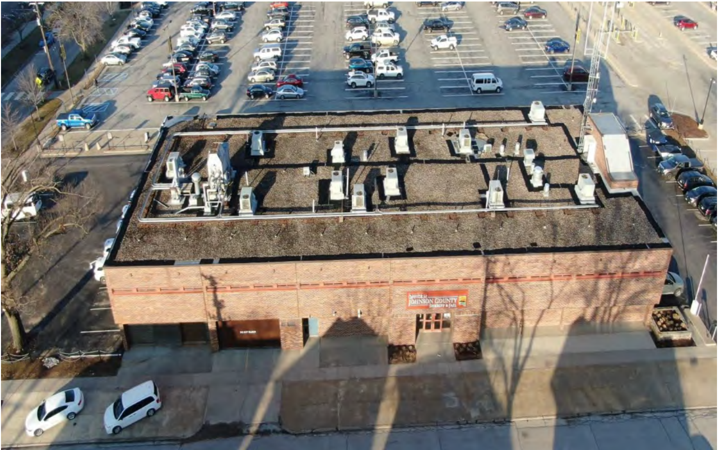
Drone image of overall building – March 2023
