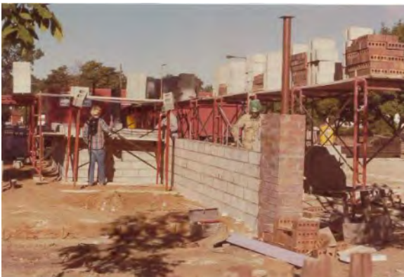
Masonry construction of lower floor
