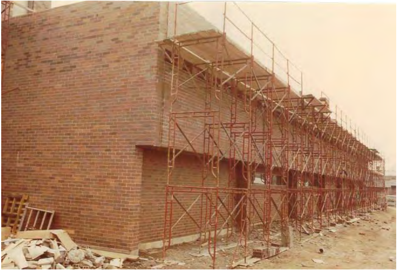
1980 construction of the cantilvered second level edge
