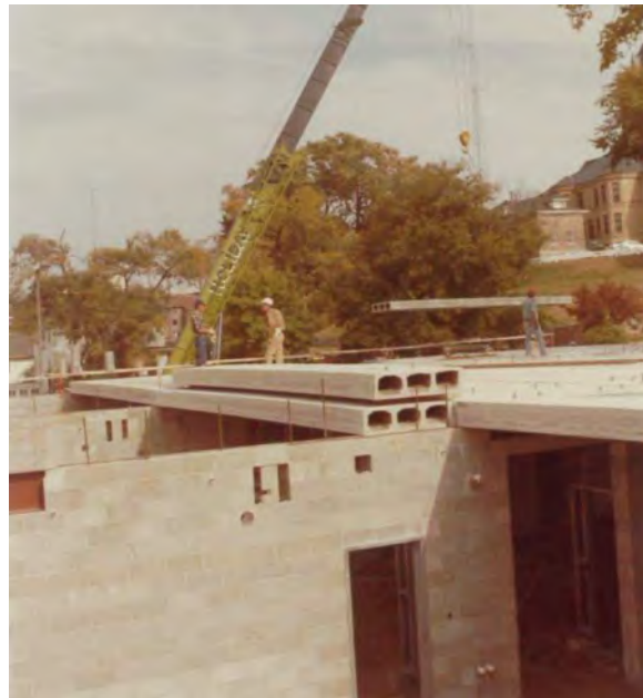
Hollowcore precast second level floor construction
