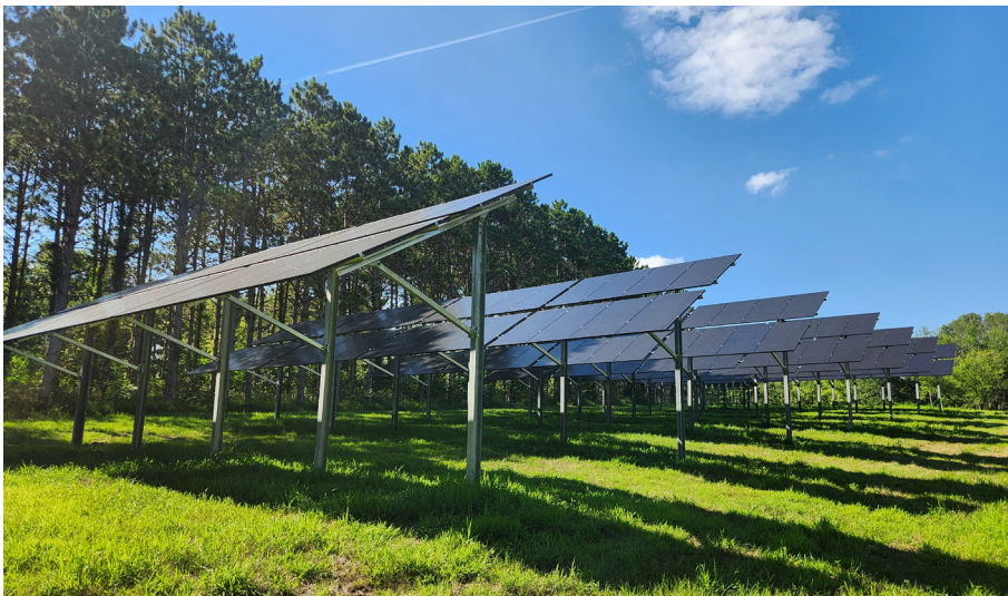
Left: The new 112.84 kW solar array at Kent Park more than doubles the energy-producing capacity of the two other arrays already in the park. Energy produced will supply park operations and park users and also enter back into the electrical grid. Right: One of the hydrology wells at Pechman Creek Delta that is being used to study ground water depth throughout the property.
