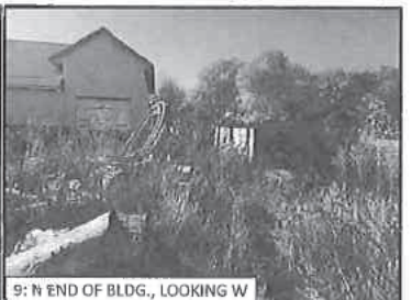
9: N END OF BLDG., LOOKING W
