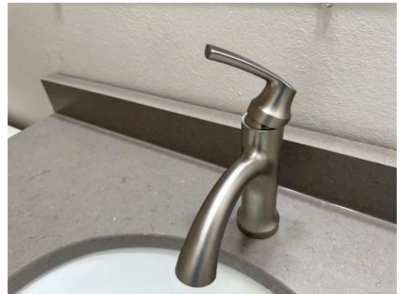
Unit # 14 Bathroom: NO WATER TO SINK
