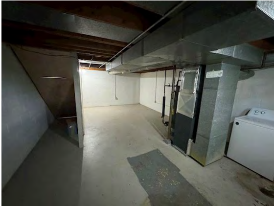
Unit # 4 Interior Foundation:
