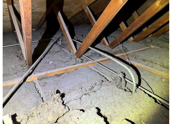
North Building Attic Insulation:
