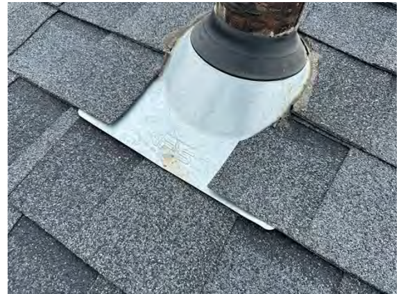
North Building Flashing/Valleys:
