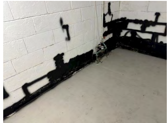
Unit # 12 Interior Foundation:
