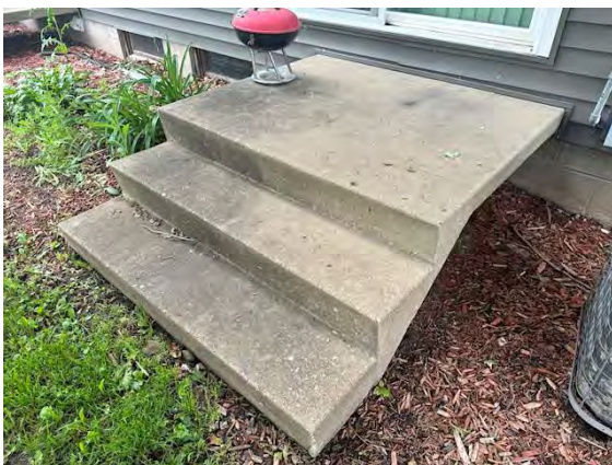
Complex Flatwork / Sidewalks:
