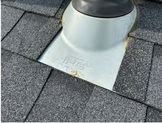
North Building Flashing/Valleys:
