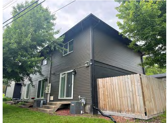
West Building Exterior Surface:
