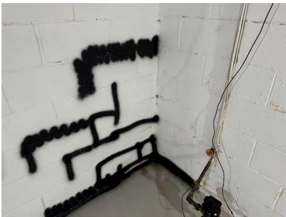
Unit # 15 Interior Foundation:
