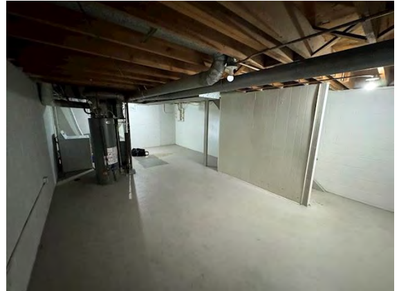
Unit # 4 Interior Foundation:
