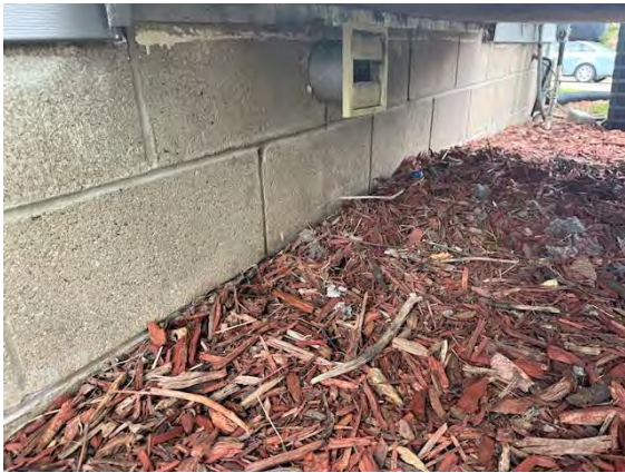
West Building Exterior Foundation:
