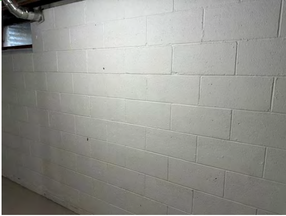
Unit # 13 Interior Foundation:
