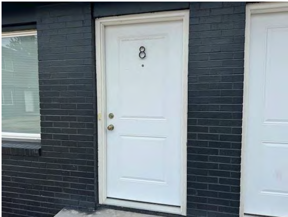
North Building Unit Main Doors:
