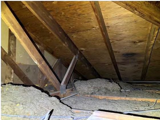
North Building Attic / Roof Framing and Sheathing:
