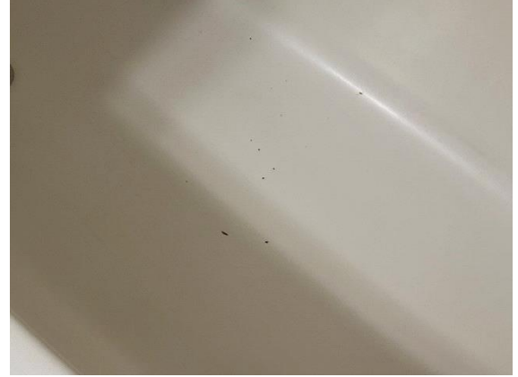
Unit # 15 Bathroom: DAMAGED TUB ENCLOSURE
