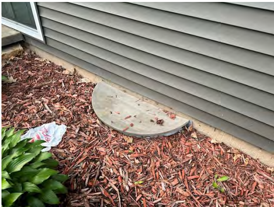
North Building Exterior Foundation:
