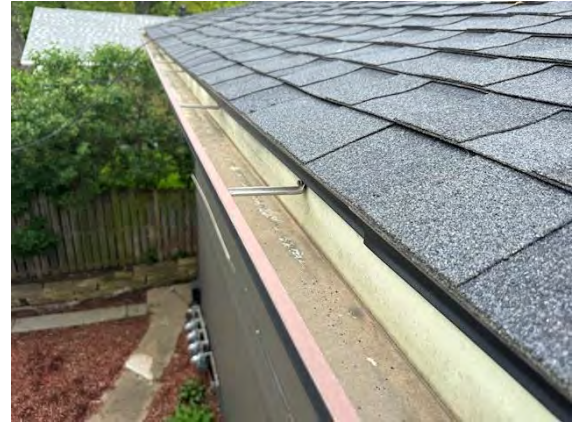
East Building Roof Drainage System:
