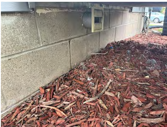
West Building Grading / Drainage:
