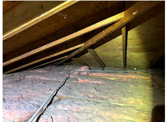
West Building Attic / Roof Framing and Sheathing:
