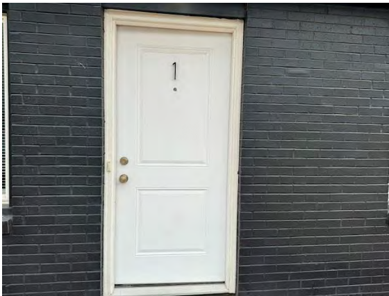
West Building Unit Main Doors:
