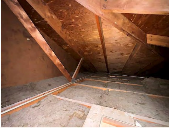
East Building Attic / Roof Framing and Sheathing:
