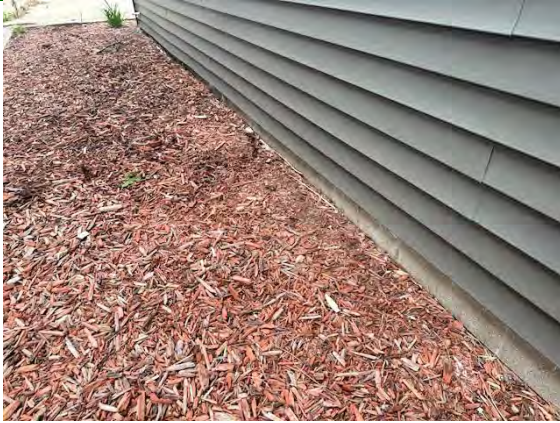
West Building Grading / Drainage:
