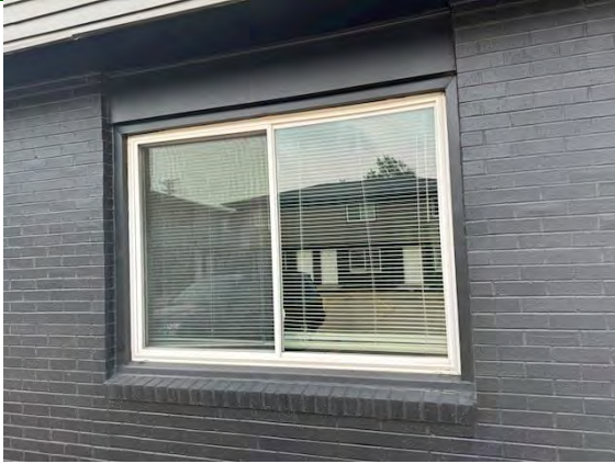
East Building Fenestration Systems:
