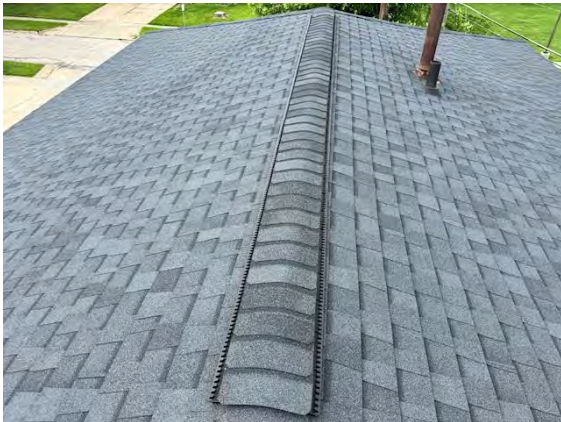
West Building Roofing:
