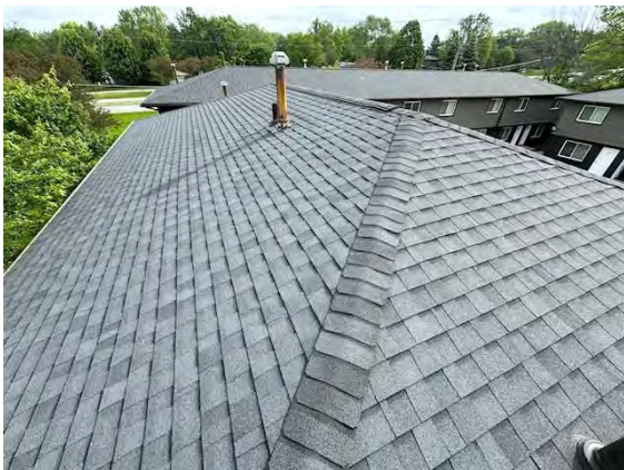
West Building Roofing:
