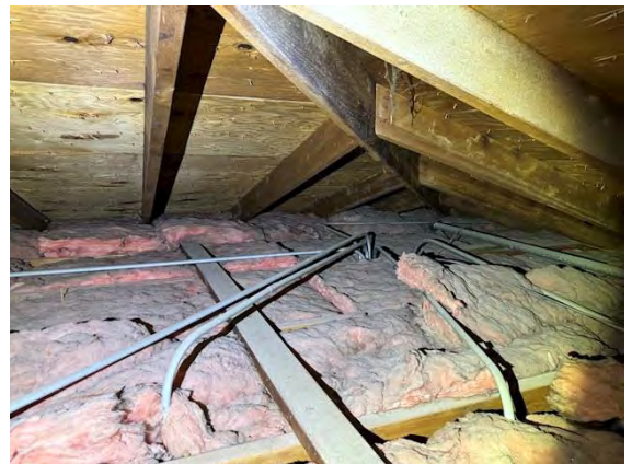
West Building Attic / Roof Framing and Sheathing:
