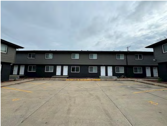
North Building Exterior Surface:
