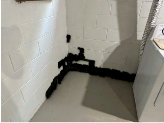
Unit # 15 Interior Foundation:
