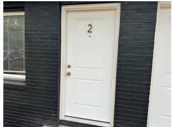
West Building Unit Main Doors:
