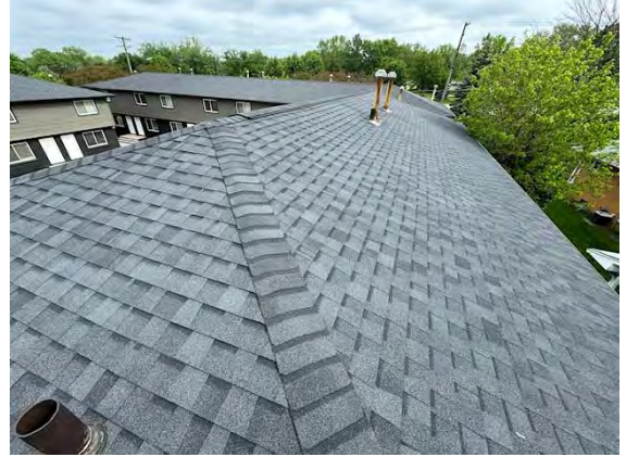
East Building Roofing:
