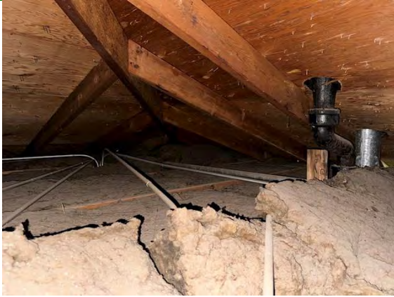
East Building Attic / Roof Framing and Sheathing:
