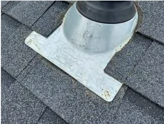
East Building Flashing / Valleys:
