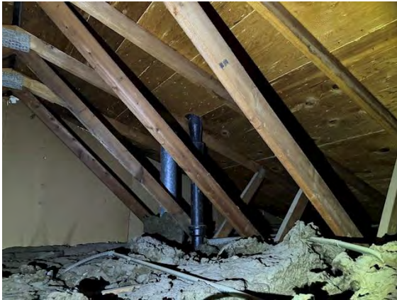
West Building Attic / Roof Framing and Sheathing:
