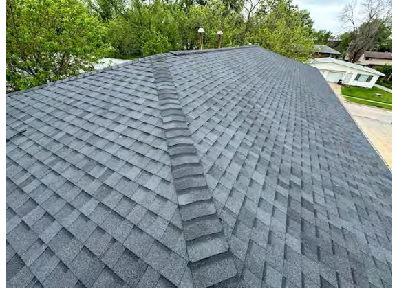
East Building Roofing:
