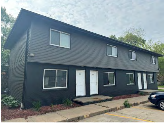
East Building Exterior Surface:
