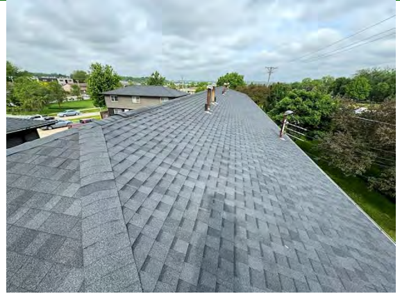
North Building Roofing:
