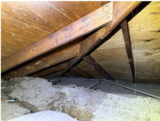
West Building Attic / Roof Framing and Sheathing:
