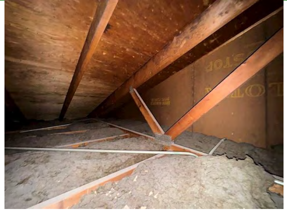
East Building Attic / Roof Framing and Sheathing:
