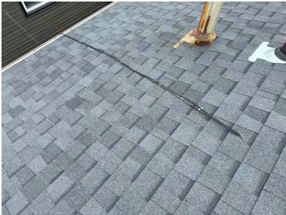
East Building Roofing: WIRE LAYING ON ROOF SHINGLES
