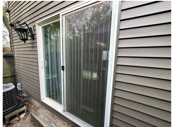
East Building Unit Patio Doors:
