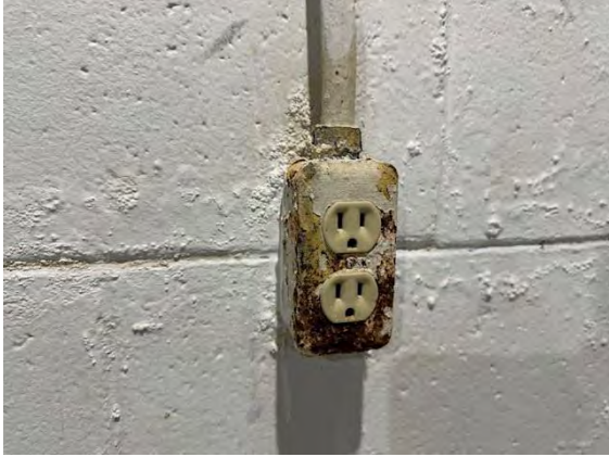
Unit # 9 Interior Foundation:
