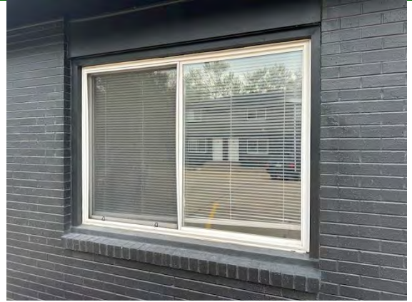
West Building Fenestration Systems:
