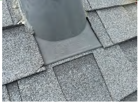
West Building Flashing/Valleys:
