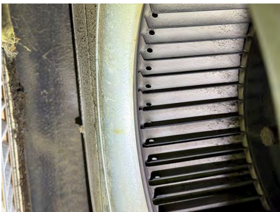
Unit # 8 HVAC Distribution:
