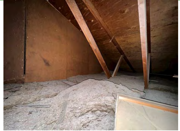
East Building Attic Insulation:
