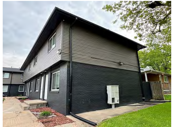
East Building Exterior Surface:
