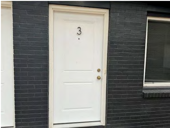
West Building Unit Main Doors:
