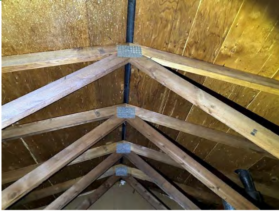
West Building Attic Ventilation:
