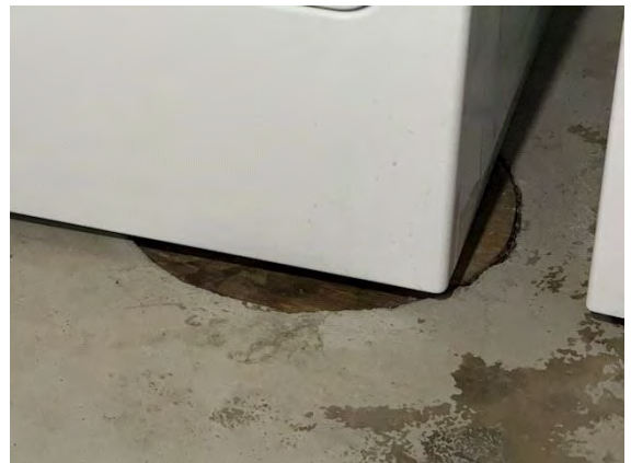
Sump/Sump Pumps Systems:
