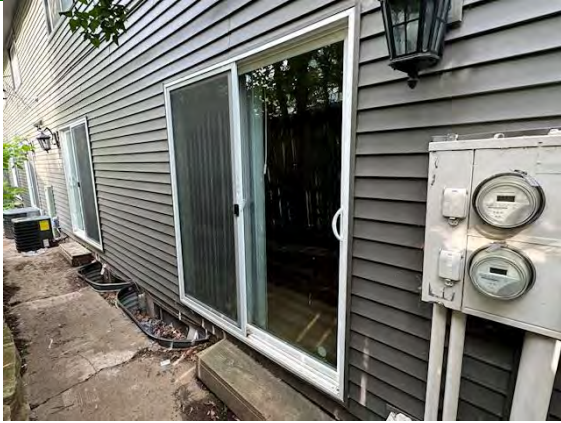
East Building Unit Patio Doors:
