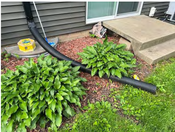
North Building Roof Drainage System:
