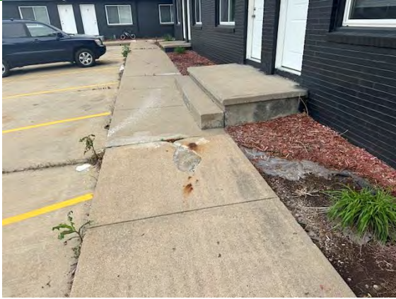
Complex Flatwork / Sidewalks:
