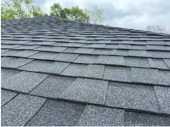
East Building Roofing:
