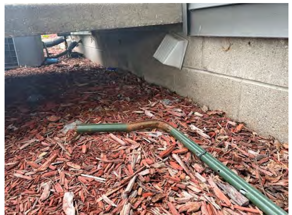
West Building Grading / Drainage:
