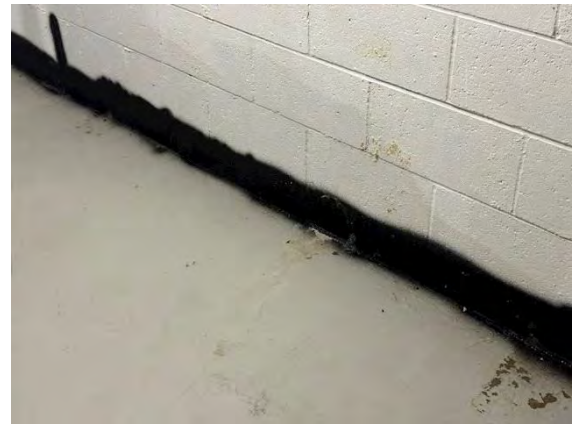
Unit # 14 Interior Foundation:
