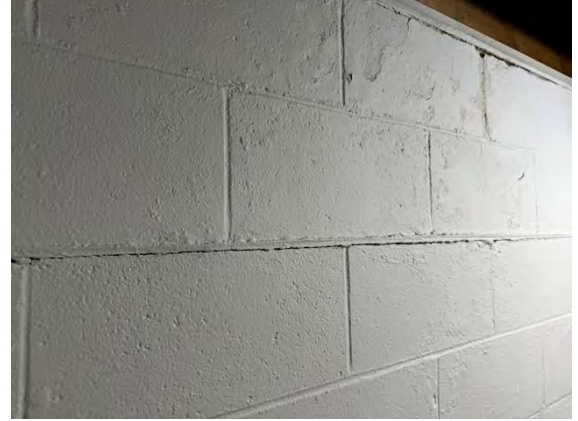
Unit # 12 Interior Foundation:
