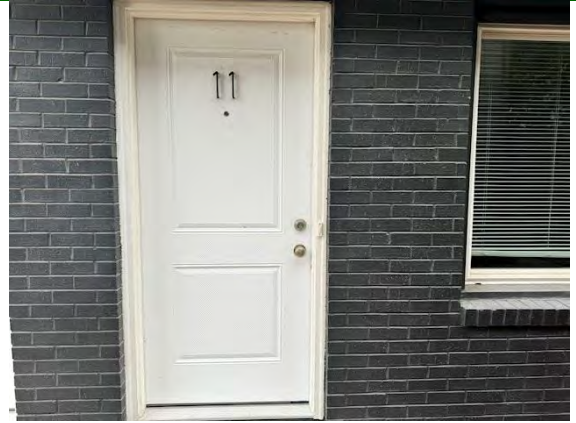
North Building Unit Main Doors:
