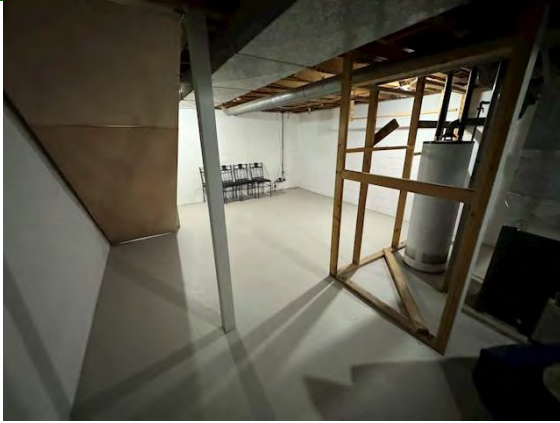
Unit # 14 Interior Foundation:
