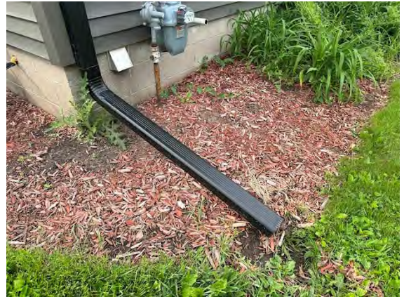
North Building Roof Drainage System:
