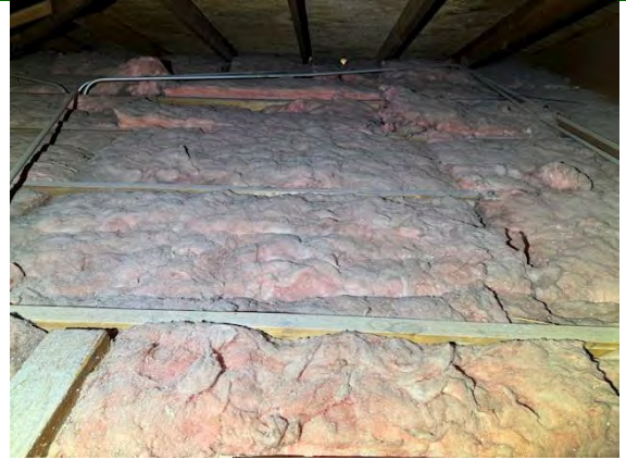
West Building Attic Insulation:
