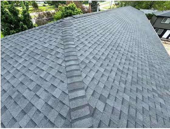
North Building Roofing:
