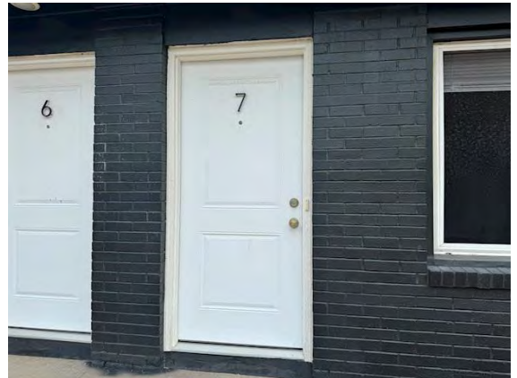
North Building Unit Main Doors:
