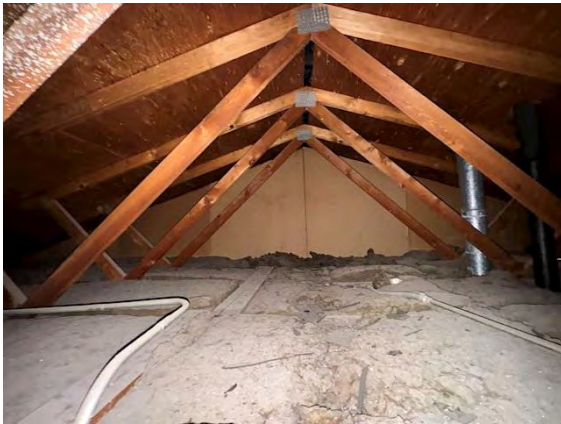
East Building Attic / Roof Framing and Sheathing:
