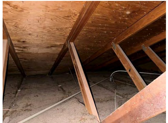
East Building Attic / Roof Framing and Sheathing:
