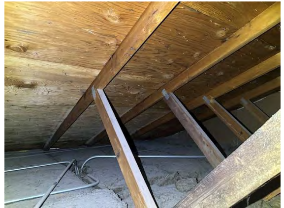
North Building Attic / Roof Framing and Sheathing:
