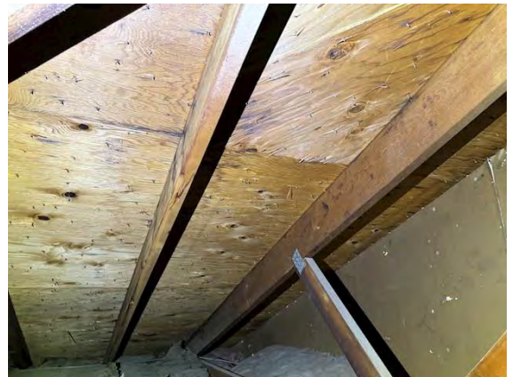
West Building Attic / Roof Framing and Sheathing:
