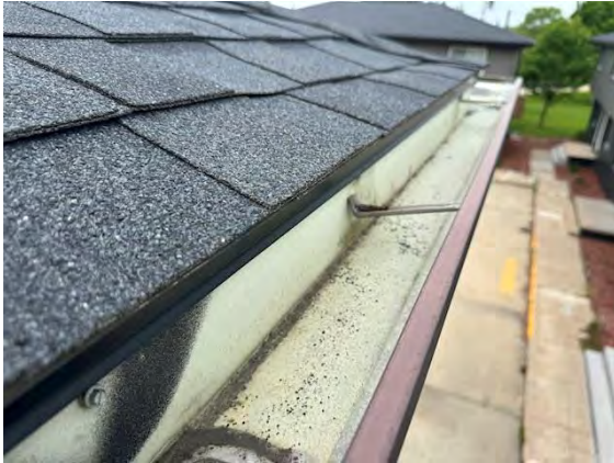
East Building Roof Drainage System:
