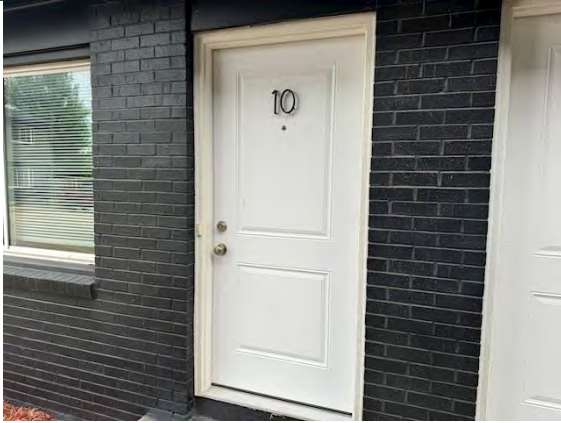
North Building Unit Main Doors:
