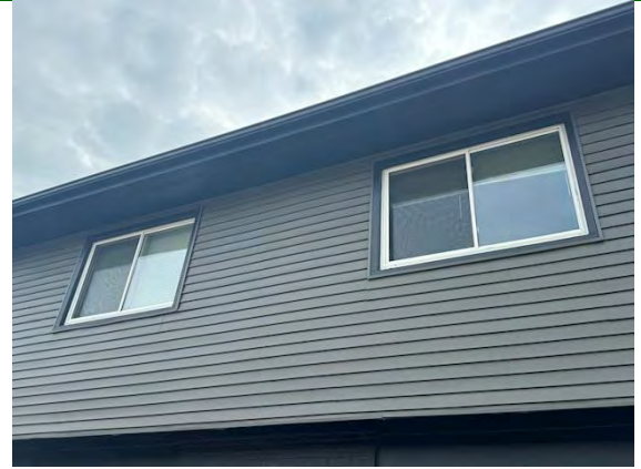
East Building Fenestration Systems:
