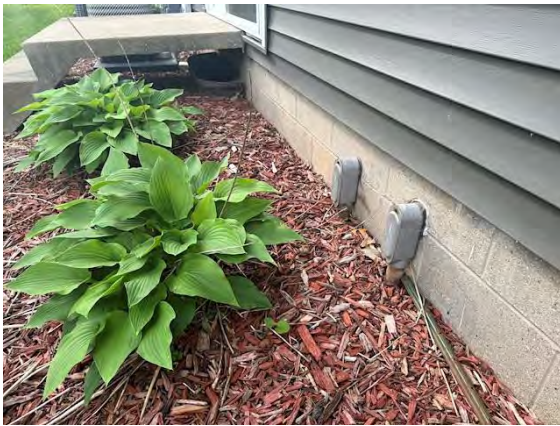
North Building Grading / Drainage:
