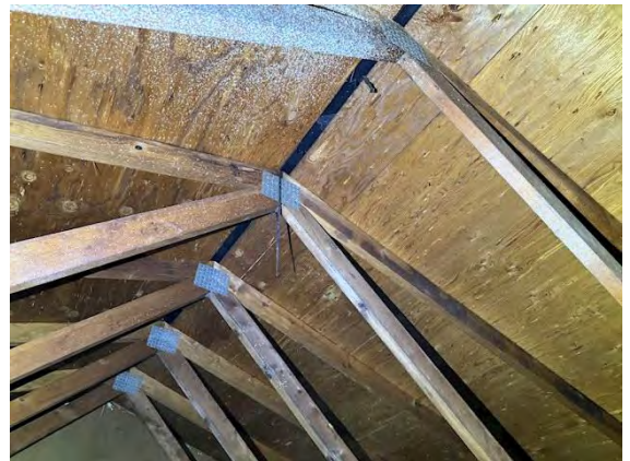
North Building Attic Ventilation:
