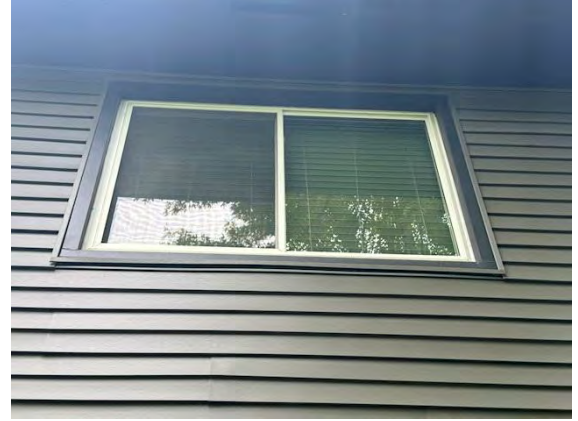
West Building Fenestration Systems:
