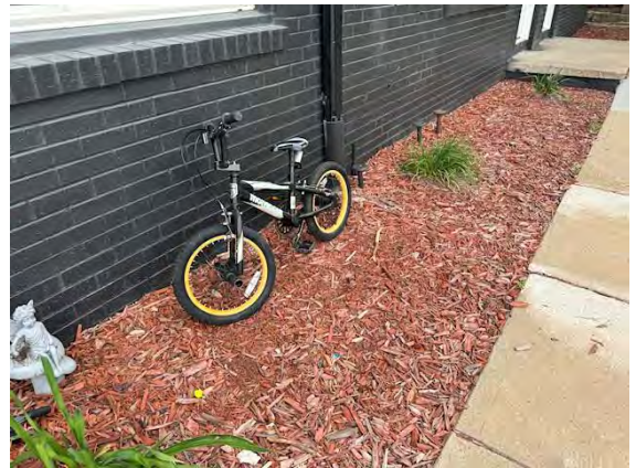
North Building Grading / Drainage:
