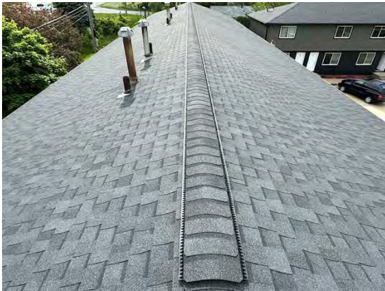
North Building Attic Ventilation:
