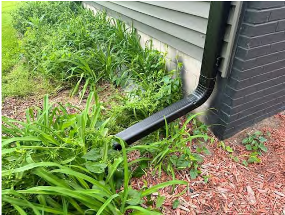
North Building Roof Drainage System:
