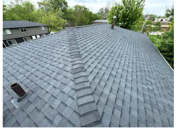
West Building Roofing:
