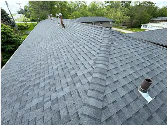
North Building Roofing:
