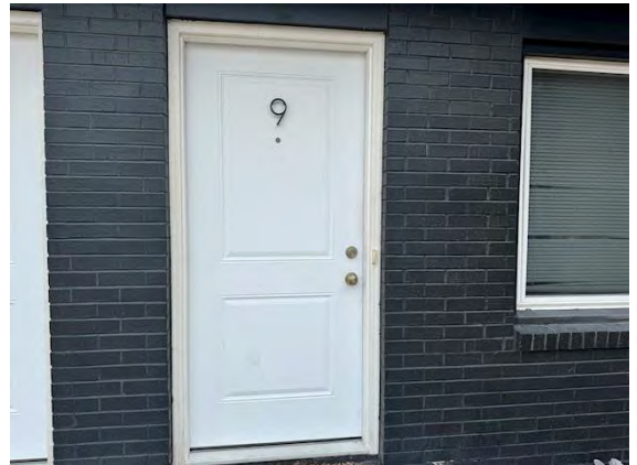
North Building Unit Main Doors:
