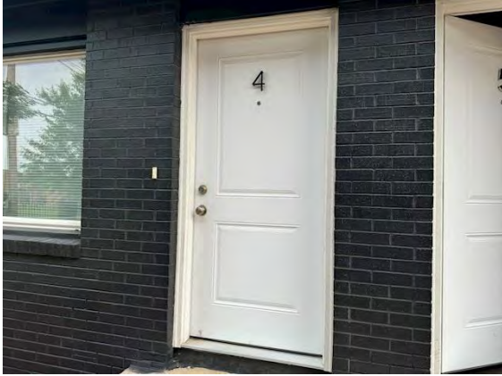
North Building Unit Main Doors:
