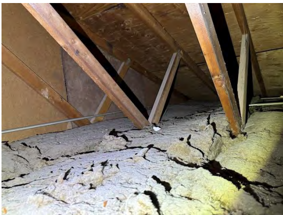
West Building Attic Insulation:
