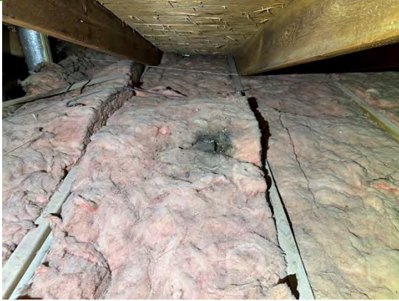
West Building Attic Insulation:
