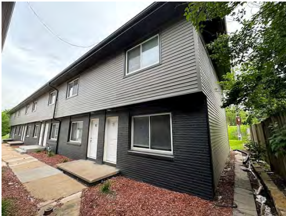
North Building Exterior Surface:
