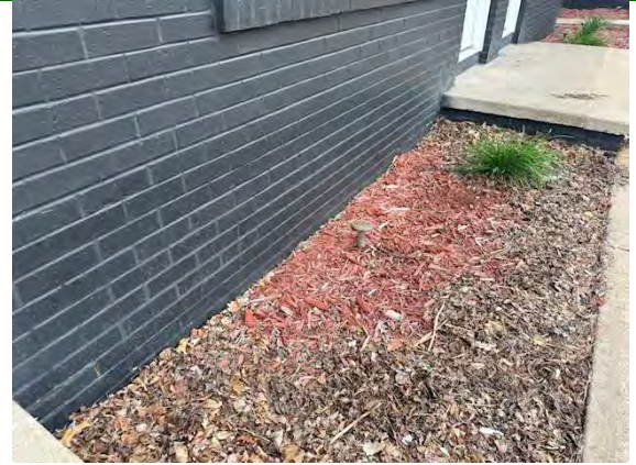
West Building Grading / Drainage:
