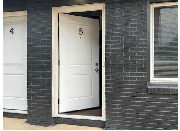
North Building Unit Main Doors:
