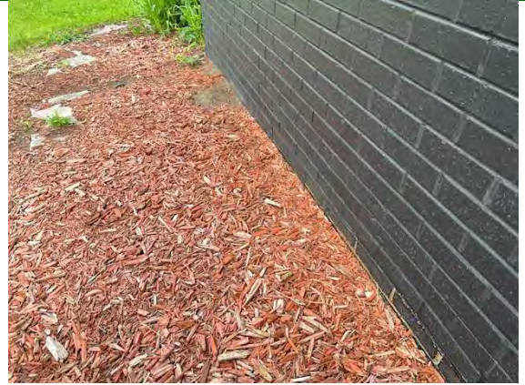
North Building Grading / Drainage:
