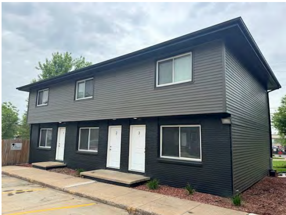
West Building Exterior Surface:
