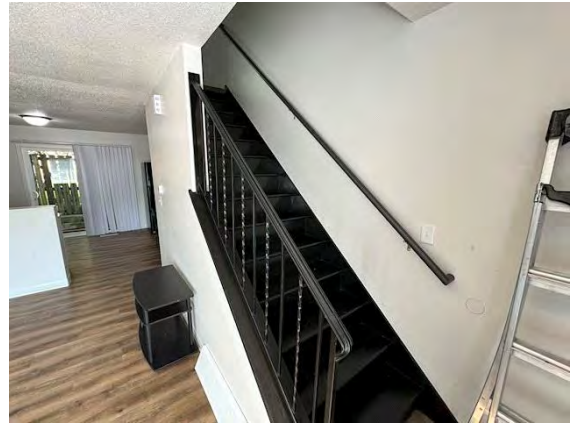
Unit # 12 Stairs / Railings:
