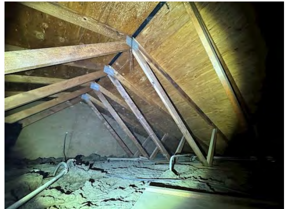
North Building Attic / Roof Framing and Sheathing:
