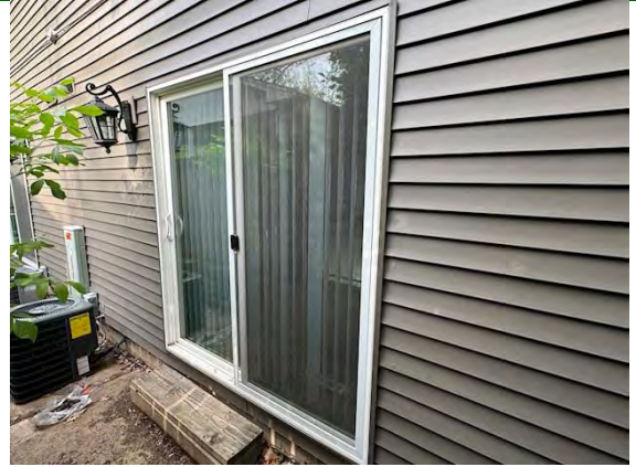
East Building Unit Patio Doors:
