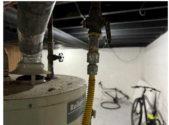
Unit # 8 Plumbing : CSST INSTALLED AT WATER HEATER
