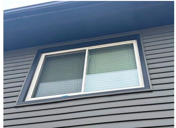
East Building Fenestration Systems:
