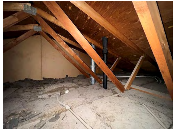
East Building Attic / Roof Framing and Sheathing:
