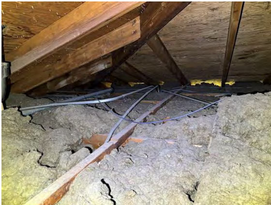
North Building Attic Insulation:
