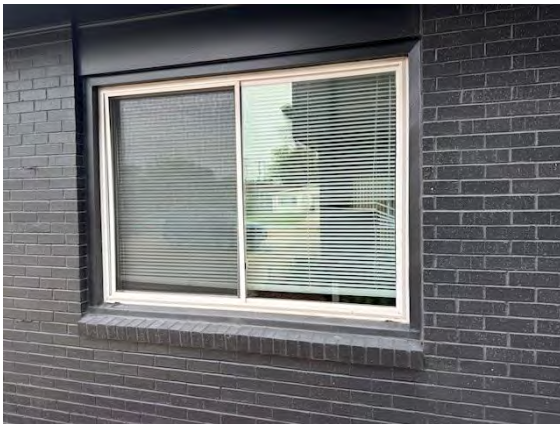
North Building Fenestration Systems:
