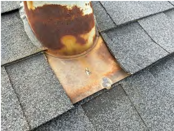
West Building Flashing/Valleys:
