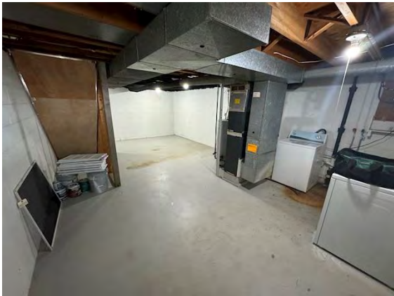
Unit # 1 Interior Foundation:
