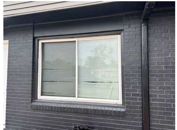
North Building Fenestration Systems:
