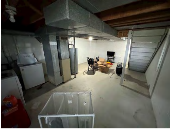
Unit # 3 Interior Foundation:
