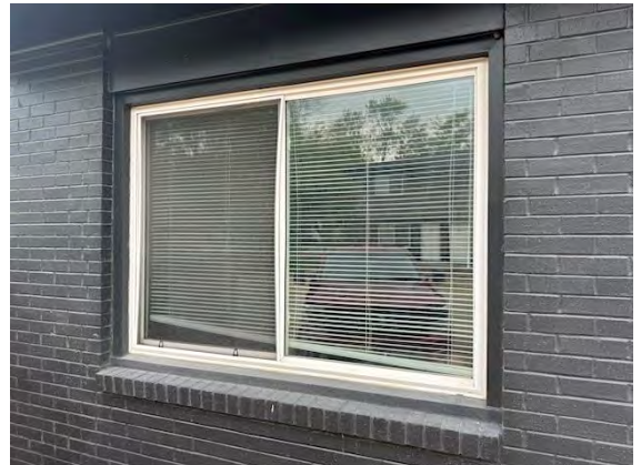
West Building Fenestration Systems:
