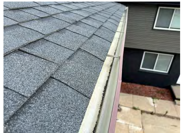
West Building Roof Drainage System:
