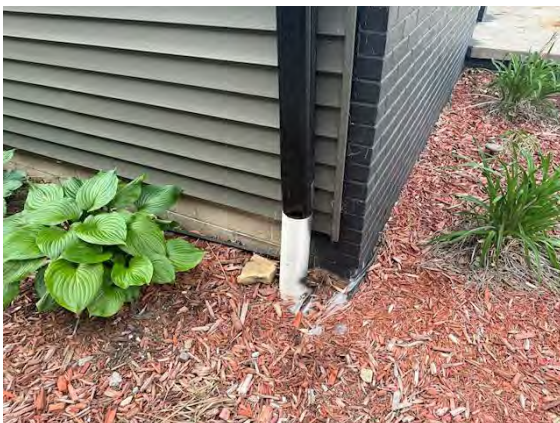
East Building Roof Drainage System:
