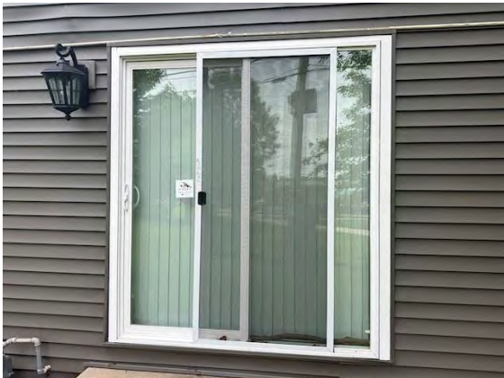
West Building Unit Patio Doors:
