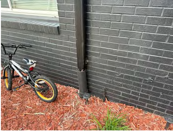
North Building Roof Drainage System:
