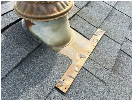
West Building Flashing/Valleys:
