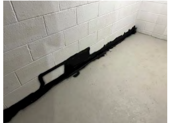
Unit # 13 Interior Foundation:
