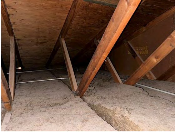
East Building Attic Insulation:
