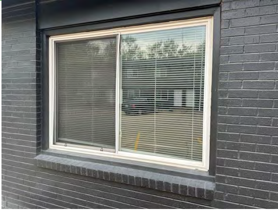
West Building Fenestration Systems:
