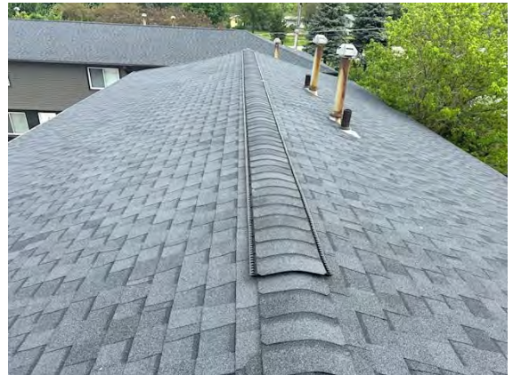
East Building Roofing:
