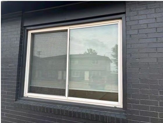
East Building Fenestration Systems:
