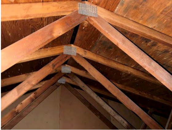
East Building Attic Ventilation:
