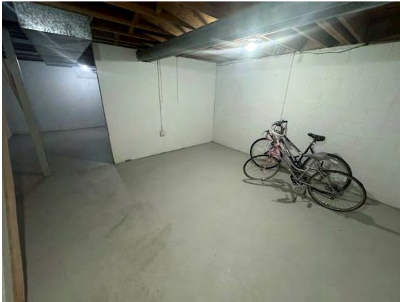
Unit # 5 Interior Foundation:
