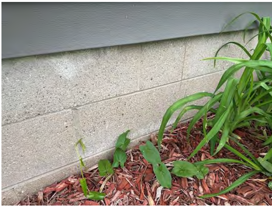
North Building Exterior Foundation:
