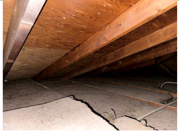
East Building Attic / Roof Framing and Sheathing:
