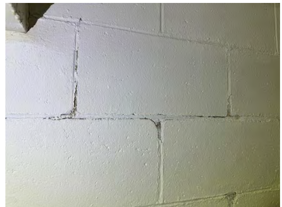
Unit # 7 Interior Foundation:
