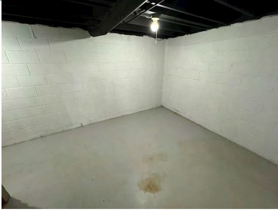
Unit # 1 Interior Foundation:
