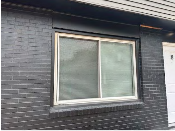
North Building Fenestration Systems:
