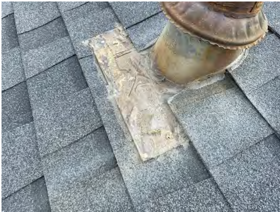
North Building Flashing/Valleys:
