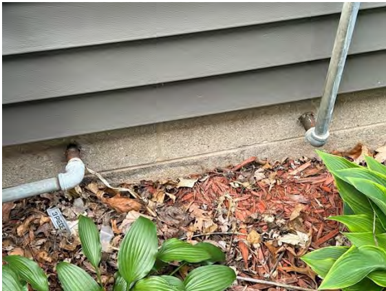
East Building Exterior Foundation: FOUNDATION PENETRATIONS
