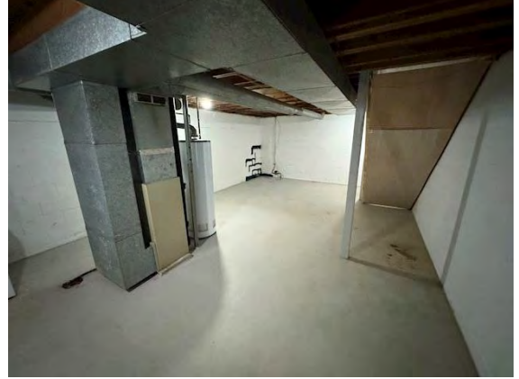
Unit # 15 Interior Foundation:
