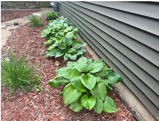
East Building Grading / Drainage:
