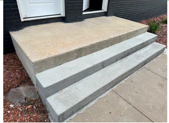
Complex Flatwork / Sidewalks:
