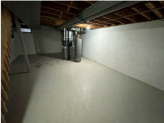
Unit # 13 Interior Foundation:
