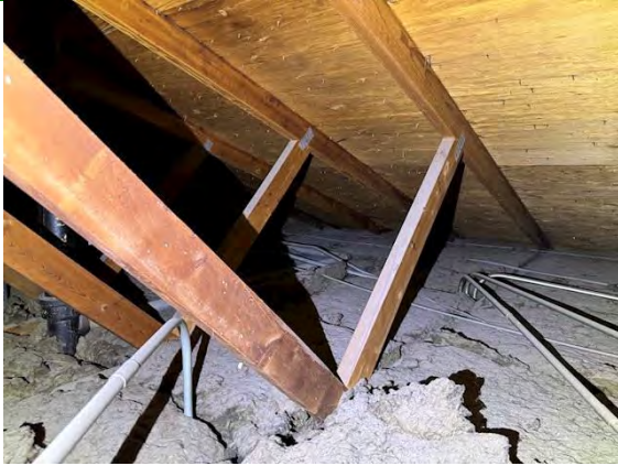
North Building Attic / Roof Framing and Sheathing:
