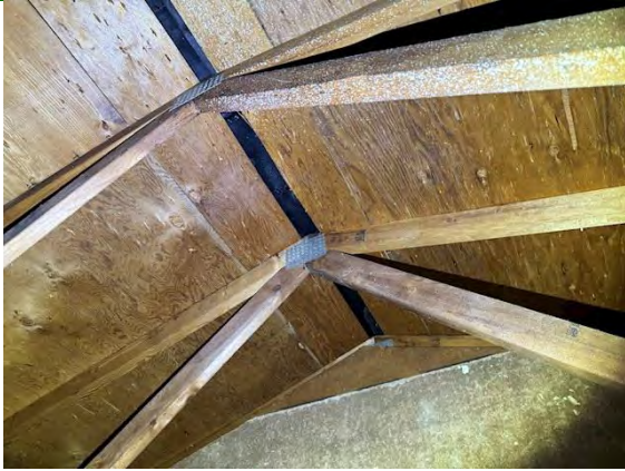
North Building Attic Ventilation:
