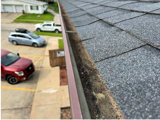
West Building Roof Drainage System:
