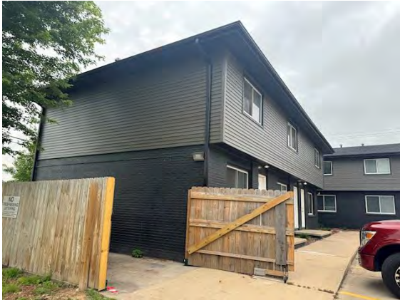
West Building Exterior Surface:
