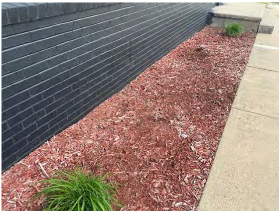
East Building Grading / Drainage:
