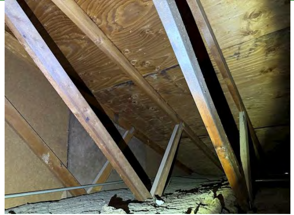
West Building Attic / Roof Framing and Sheathing:
