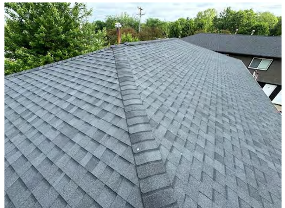
West Building Roofing:
