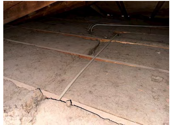
East Building Attic Insulation:
