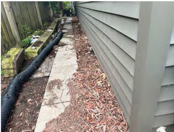
North Building Grading / Drainage:
