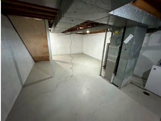
Unit # 2 Interior Foundation:
