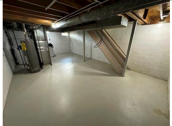
Unit # 2 Interior Foundation:
