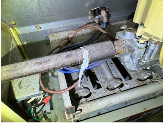
Unit # 6 Furnace: GAS CONNECTION REPAIR WITHIN FURNACE UNIT
