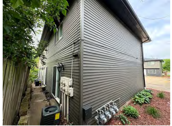
East Building Exterior Surface:
