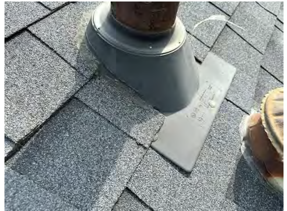
West Building Flashing/Valleys:
