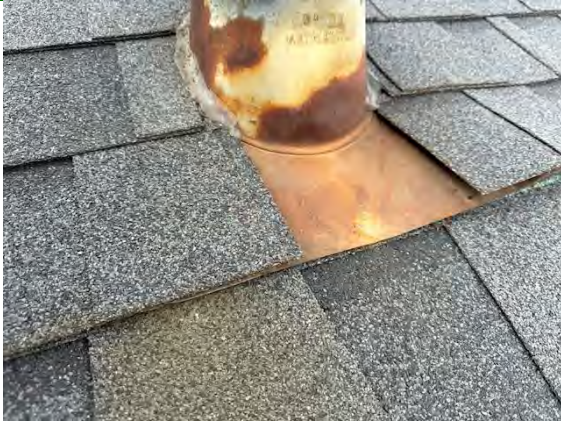
West Building Flashing/Valleys:
