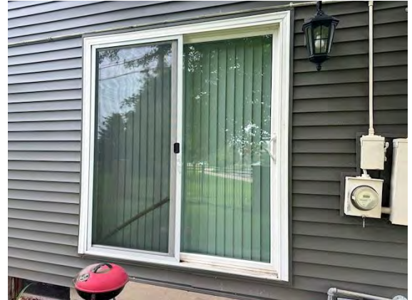
West Building Unit Patio Doors:
