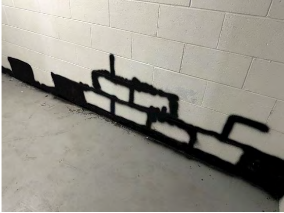
Unit # 8 Interior Foundation:
