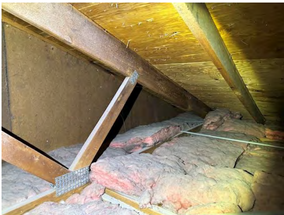
West Building Attic / Roof Framing and Sheathing:
