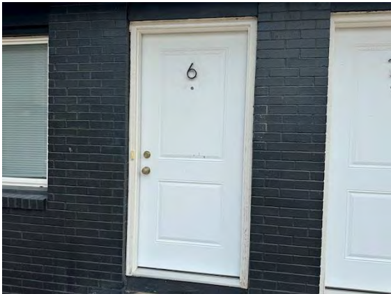
North Building Unit Main Doors:
