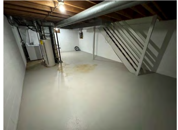
Unit # 6 Interior Foundation:
