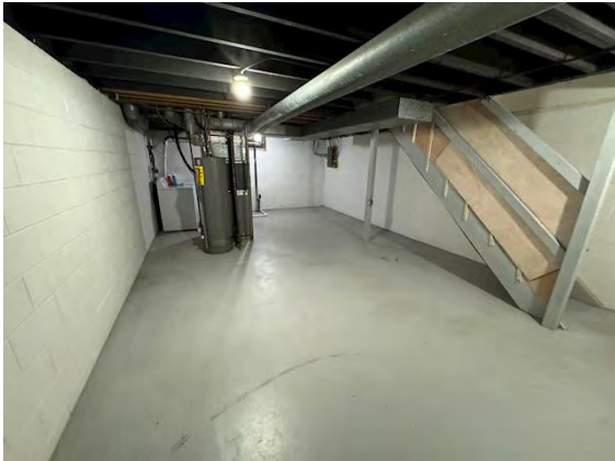
Unit # 10 Interior Foundation:
