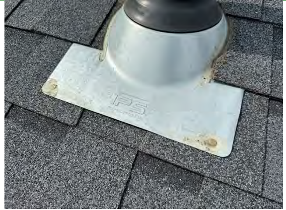
North Building Flashing/Valleys:
