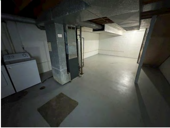
Unit # 7 Interior Foundation:
