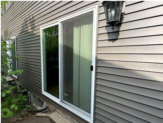
East Building Unit Patio Doors:
