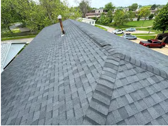
East Building Roofing:
