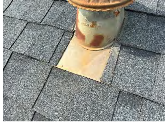
North Building Flashing/Valleys:
