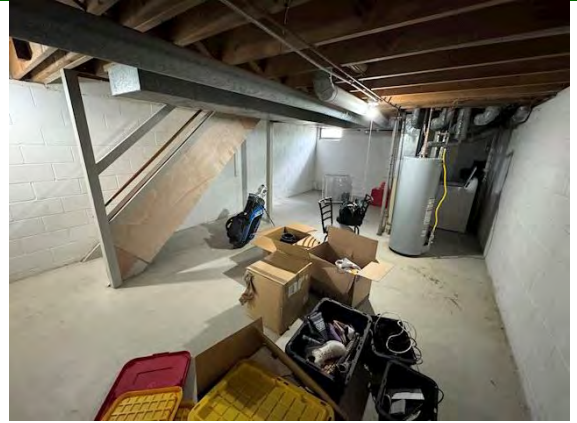
Unit # 3 Interior Foundation:
