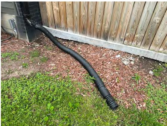
West Building Roof Drainage System:
