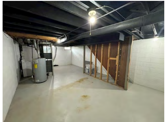
Unit # 1 Interior Foundation:
