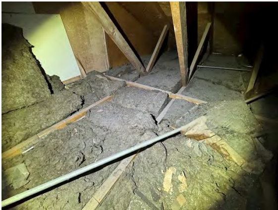
North Building Attic Insulation:
