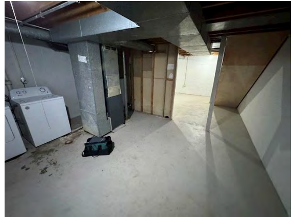
Unit # 5 Interior Foundation:
