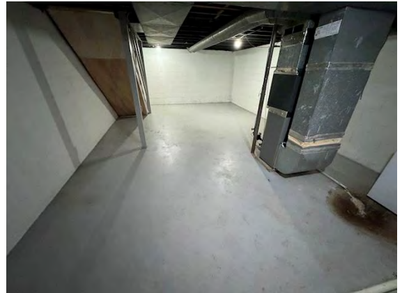
Unit # 10 Interior Foundation:
