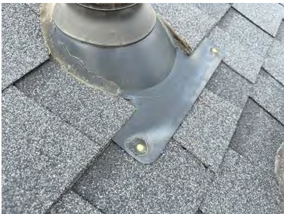
West Building Flashing/Valleys:
