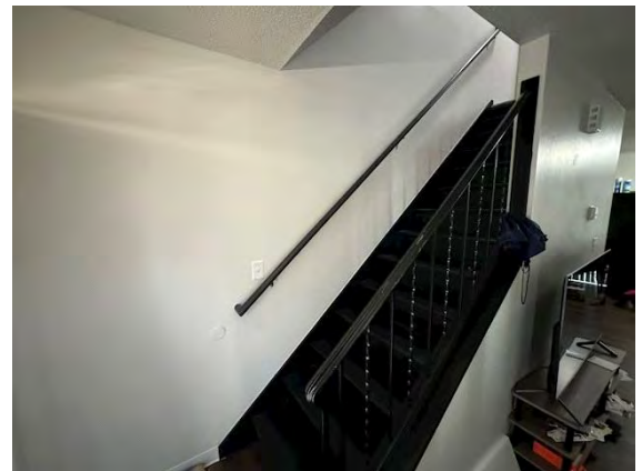
Unit # 3 Stairs / Railings:
