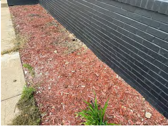
North Building Grading / Drainage:
