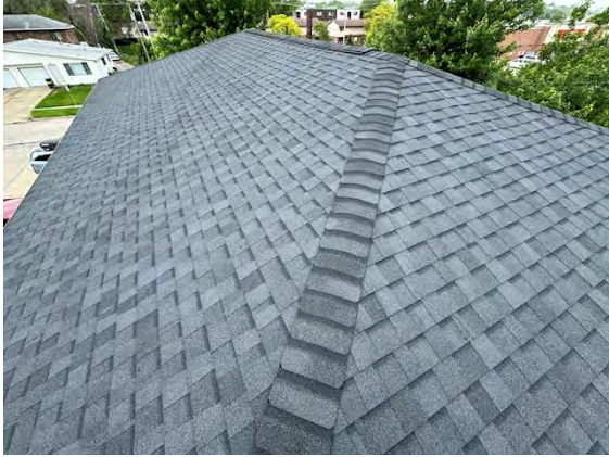
West Building Roofing:
