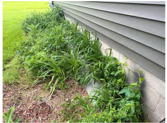
North Building Grading / Drainage:
