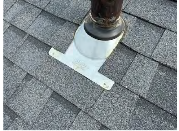
East Building Flashing / Valleys:
