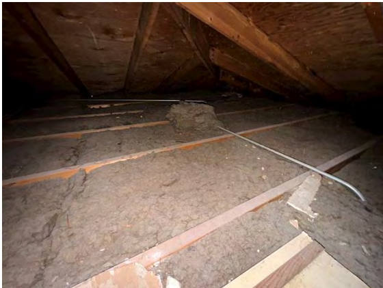
East Building Attic Insulation:
