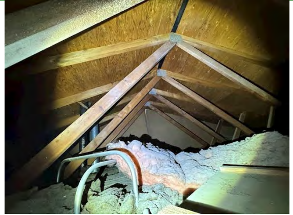
North Building Attic / Roof Framing and Sheathing:
