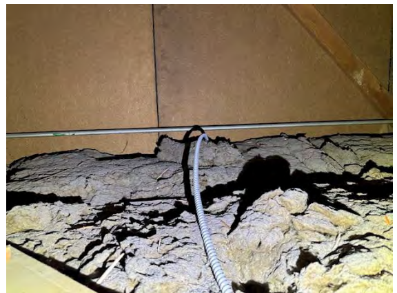
West Building Attic Insulation:
