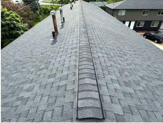
North Building Roofing:
