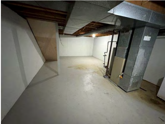
Unit # 6 Interior Foundation:
