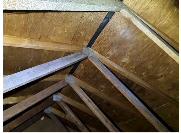
North Building Attic Ventilation:
