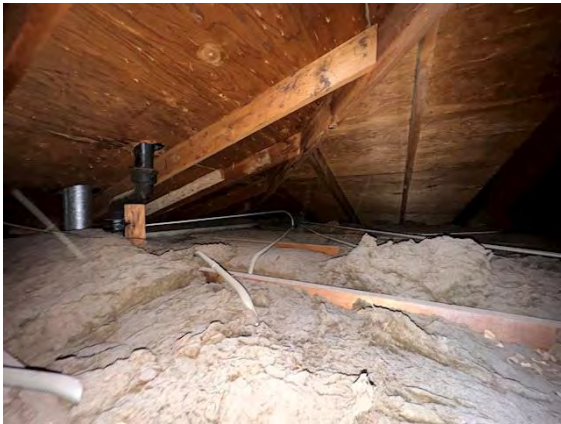
East Building Attic / Roof Framing and Sheathing:
