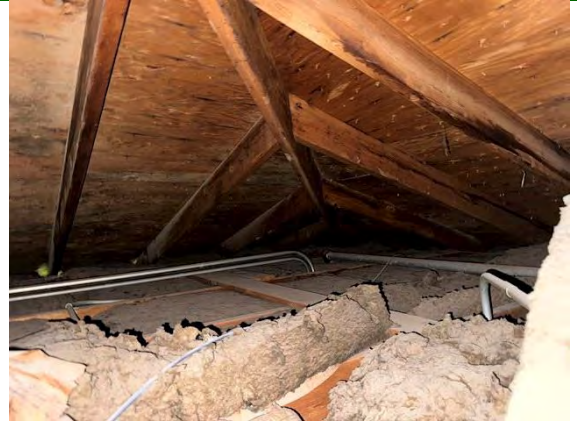
North Building Attic / Roof Framing and Sheathing:
