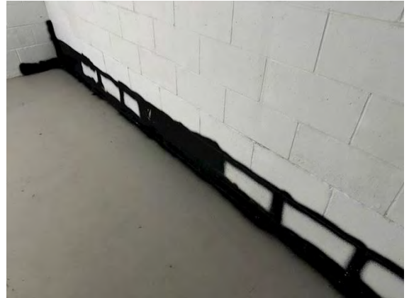
Unit # 11 Interior Foundation:
