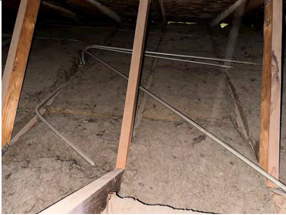
North Building Attic Insulation:
