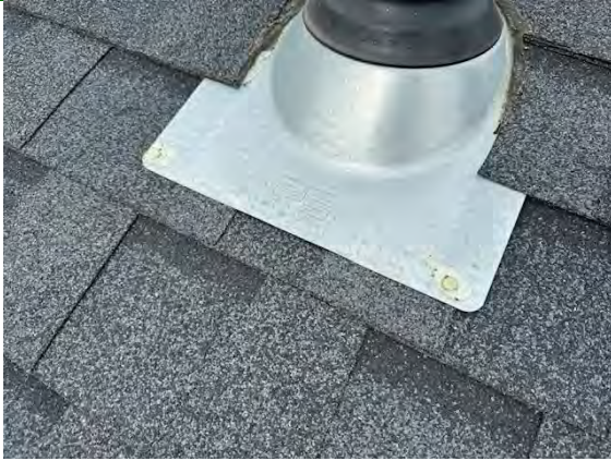
East Building Flashing / Valleys:
