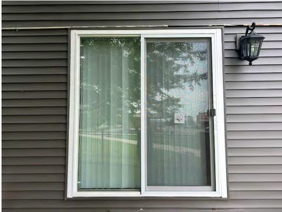
West Building Unit Patio Doors:
