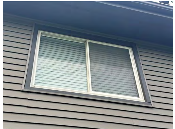
North Building Fenestration Systems:
