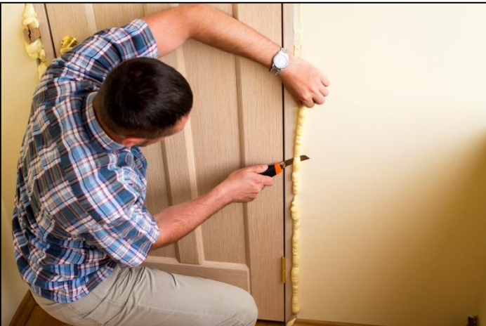
Tightly sealing openings
