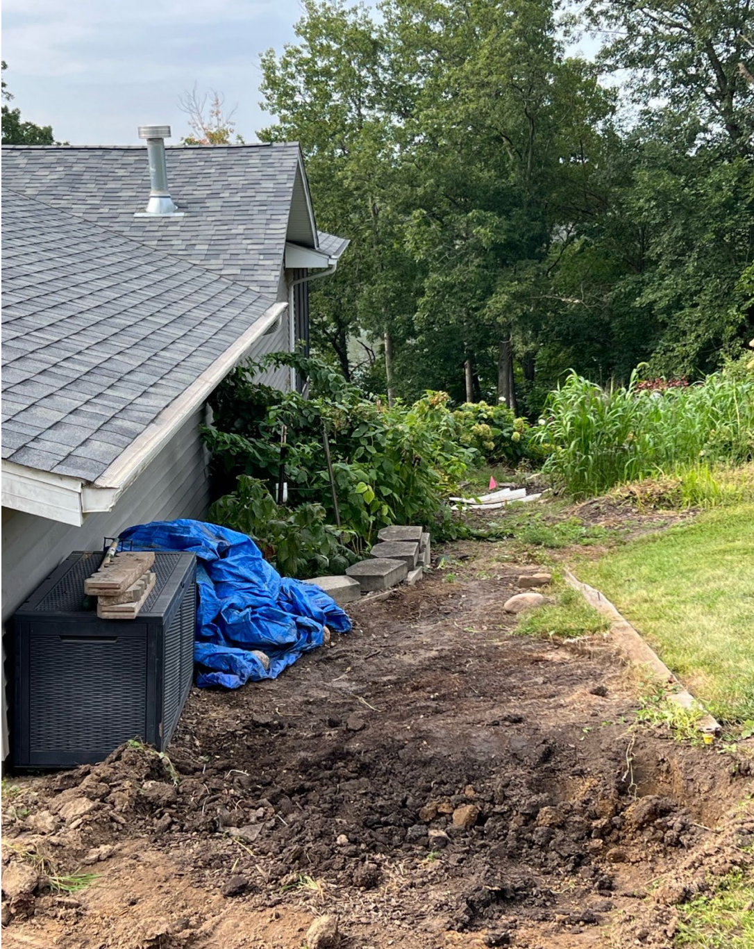
PICTURE # 4: East side yard – view from corner of the garage to back yard. The wood log on the right is the lot line .... extending down to the flag seen. This is 8' 3" from side of garage. (I recently purchased this land from the neighbor to satisfy setback requirements and clear my title.) As can be seen, no way to locate a shed. (This is a mess as I'm having work done to abate water runoff from the house above mine. Back in 2004, we put two retaining walls and drainage tiles in alongside our garage to abate water runoff from the house above us. Drain tiles are filled with dirt so redoing it to make a proper slope and trough.)
